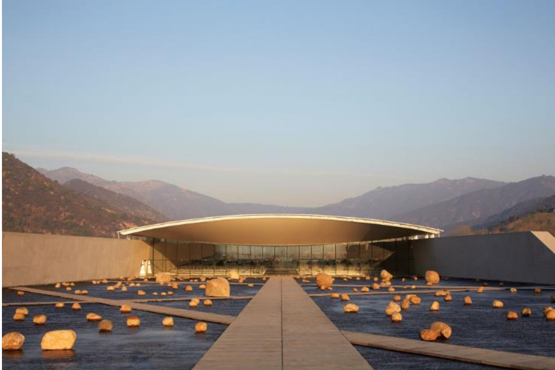
The wine is stored in large steel tanks in the catacombs beneath the forecourt, the flowing water above provides additional cooling. Photo © Cristobal Palma
