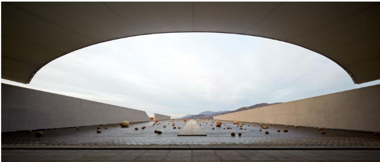
The main building rises up, whereby the interior is suffused with natural light thanks to the translucent fabric used to span the bright, curved roof. Photo © Cristobal Palma
